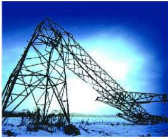
Collapse of Transmission Towers during Haiti Earthquake
