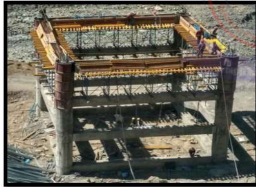
Fig 22. Scaffolding Installation
