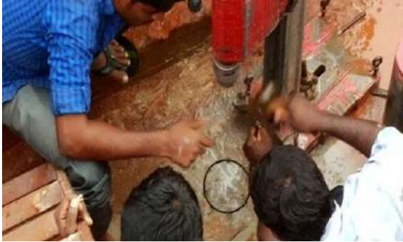
Core cutting work is completed
