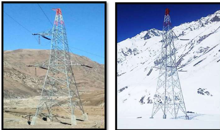
Fig 3. 220 kV S/C SINGLE ACSR DEER T.T. 'D' with cross arm staggering
