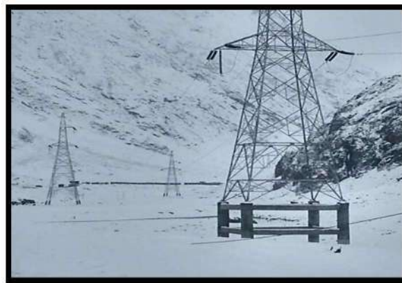
Fig 5. Raised Chimneys for increased clearance for conductors
