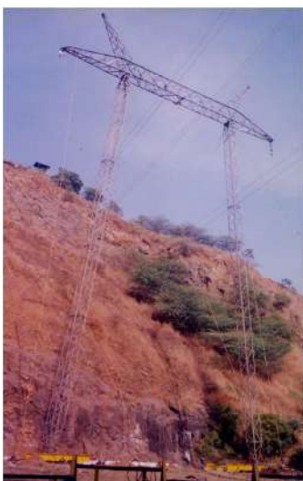
400 KV and 800 KV S/C Portal and 'V' Type Guyed Towers Testing & Analysis for First Time in India
