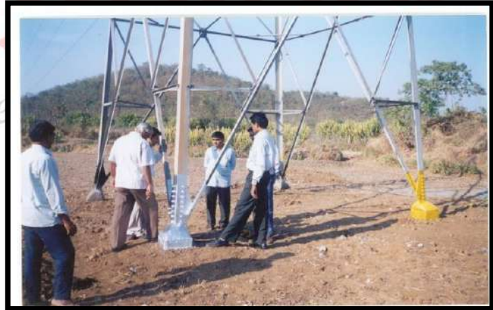
Rectification of Corroded Tower Stub using RPL Patented Stub Strengthening Technology
