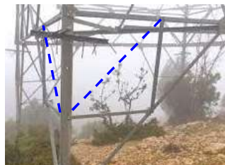
Missing Redundant Members observed during PILOT Audit
