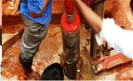
Removal of Core from the slab
