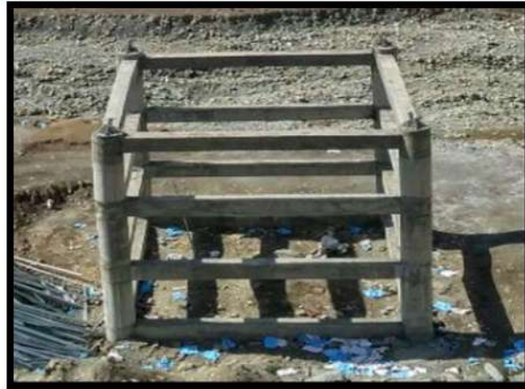
Fig 4. Special Foundation with Circular straight pedestals and tie beams
