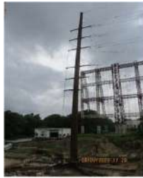
7 . Pole Type: PMT30 (15° - 30°) _21M BXA
