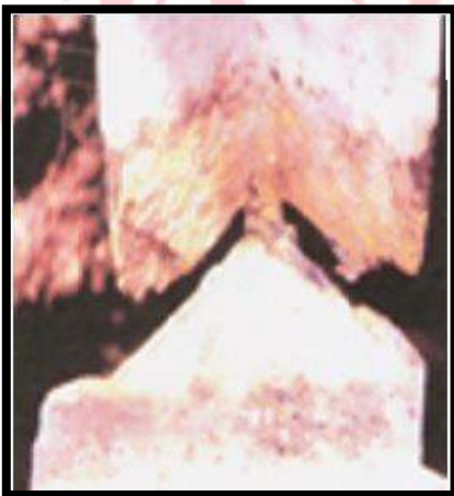
Rectification of Corroded Tower Stub using RPL Patented Stub Strengthening Technology
