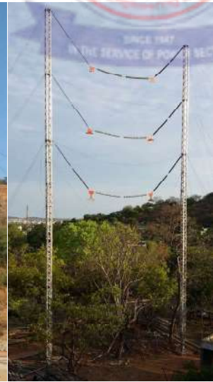
ERS for 400 kV D/C Tower
