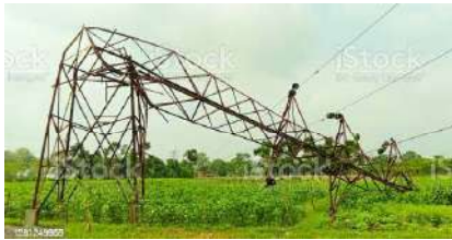
Electric tower damage during Amphan Cyclone
