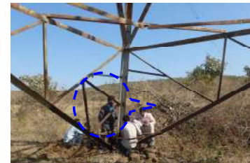
Missing Redundant Members observed during PILOT Audit
