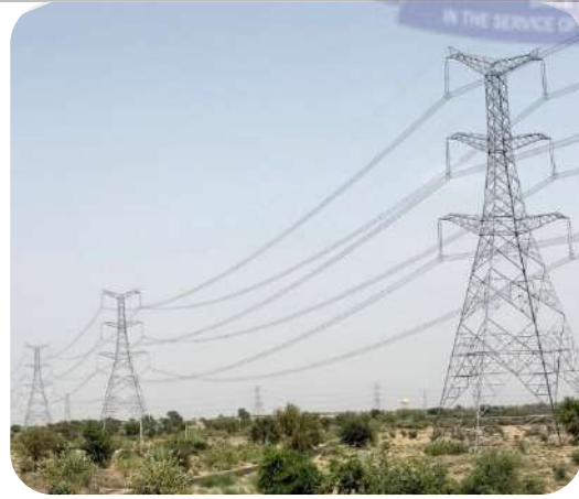
New Design of 765 kV – 20% Reduction in Weight
