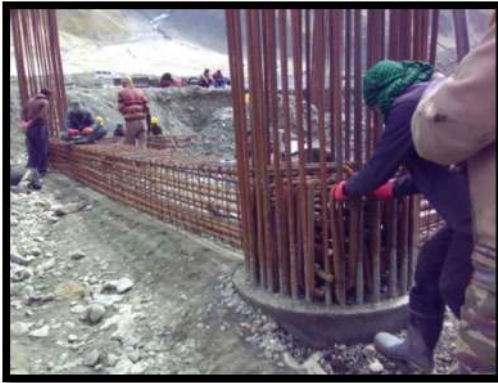
Fig 21. Reinforcement bar tying
