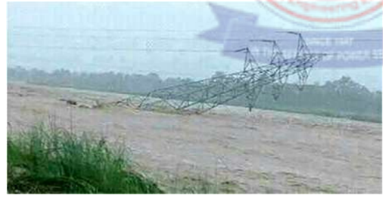
Tower Collapse in flood-hit eastern Terai, India
