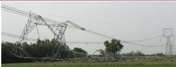
765 kV S/C Meerut-Greater Noida TL on 13.06.2016 (Tower at Location No. 464 (A+3))-Redundant member missing
