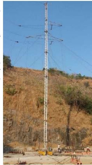
ERS for 220 kV S/C Tower
