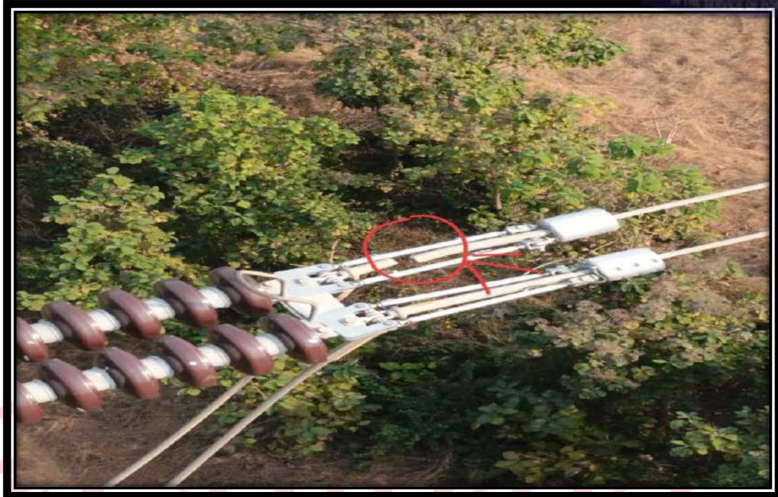
Universal Dead End Saver Clamp Assembly suitable for conductor dia. 28mm to 32mm upto 765 kV
