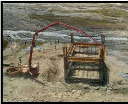
Fig 23. Casting of foundation
