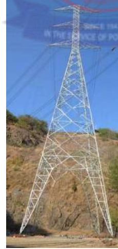
Highest D/C Tower 80 m M/s Inter Chile
